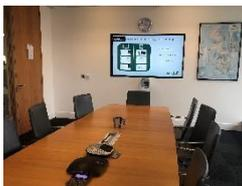
projector. Each site was then kitted out with Shure microphones and Bose speakers. Audio mixing was done using the Extron DMP products. All of the kit was then controlled by a Crestron touch panel so that a simple interface was available. This was the same set-up at both sites so users could easily move between sites confident that they could use the system with ease. For the board room, smaller rooms and
